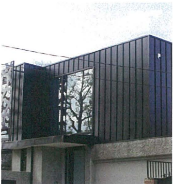
MCC1 - Metal sheet wall cladding
