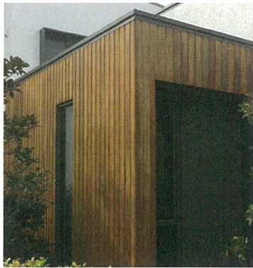
TMC - External Timber Wall Cladding
