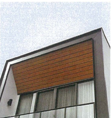
TMS - External Timber Soffit
